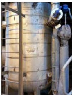
Leveraging GWR technology on blowdown flash tank for energy and condensate recovery
